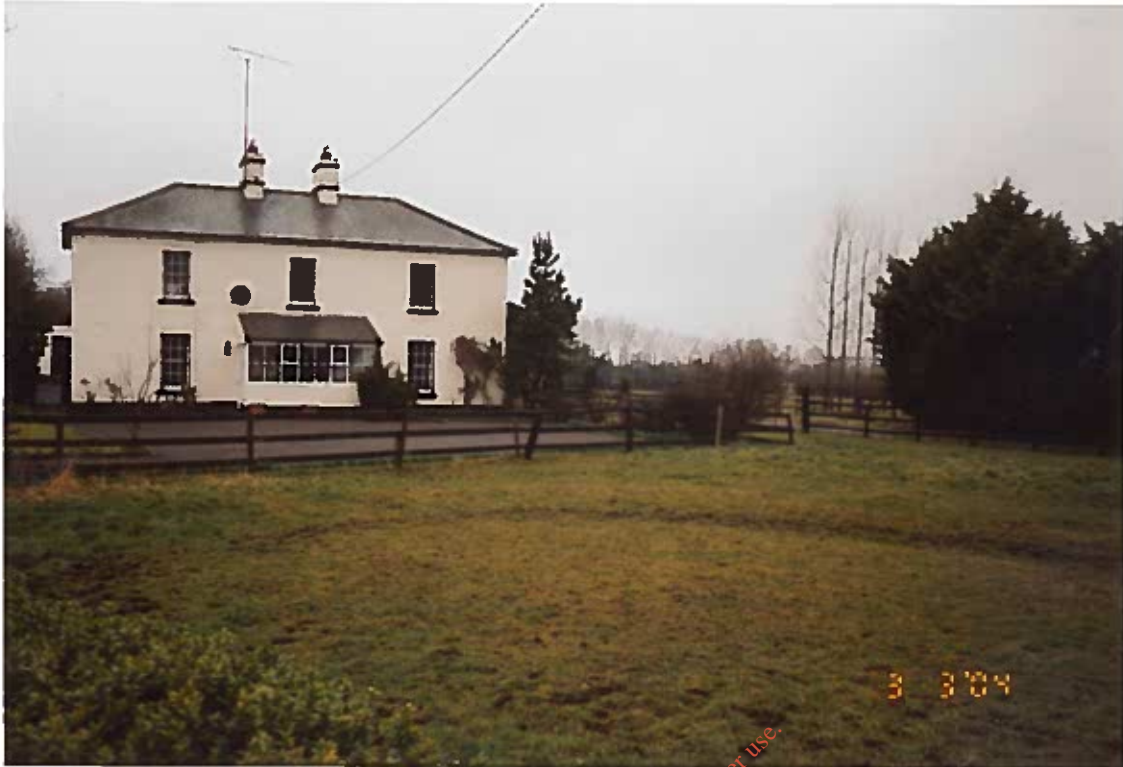
KILCANDRICK HOUSE WITH EVIDENCE OF HORSE EXERCISING IN FOREGROUND
