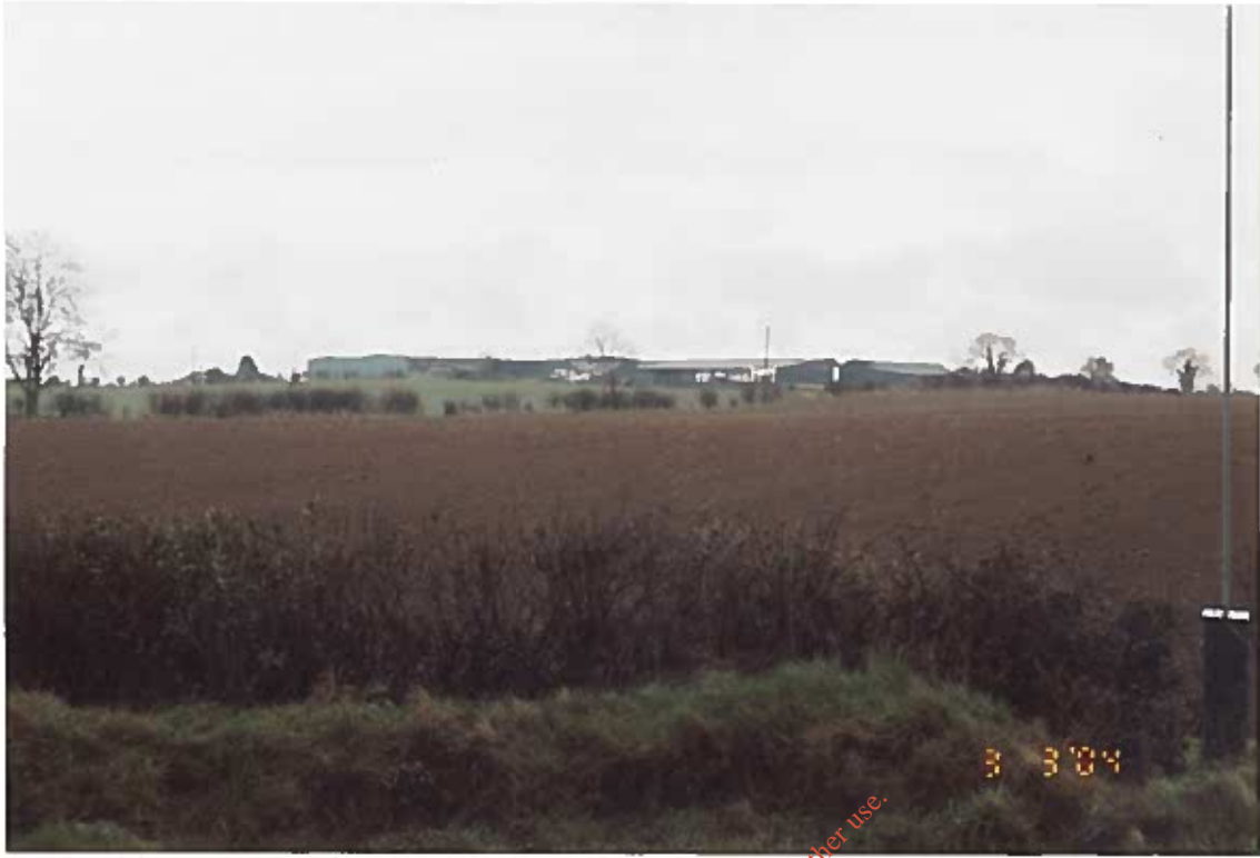
INDUSTRIAL PREMISES OF M.J. BERGIN C. 500 METRES EAST OF APPEAL SITE.
