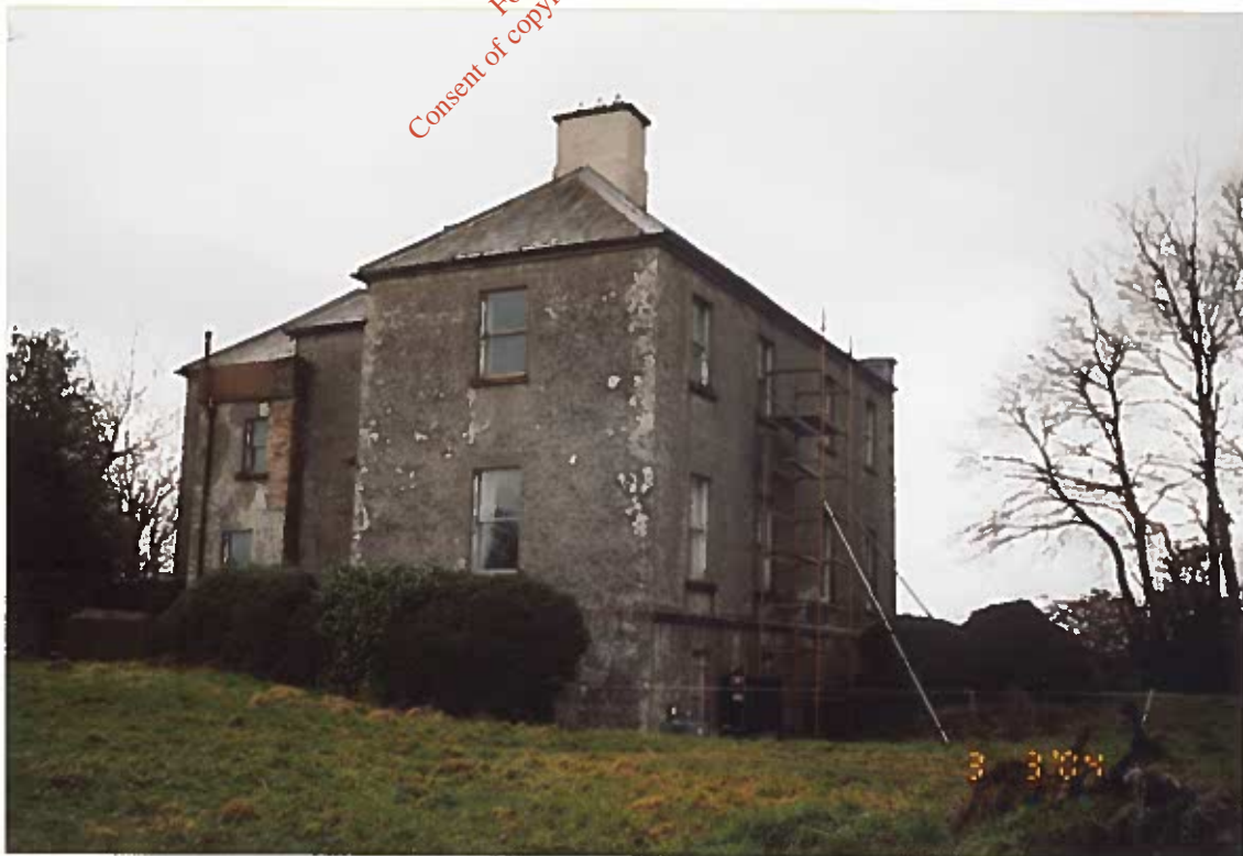
BALLINDERRY HOUSE REAR (LEFT) AND SIDE (RIGHT - WEST) ELEVATIONS.
