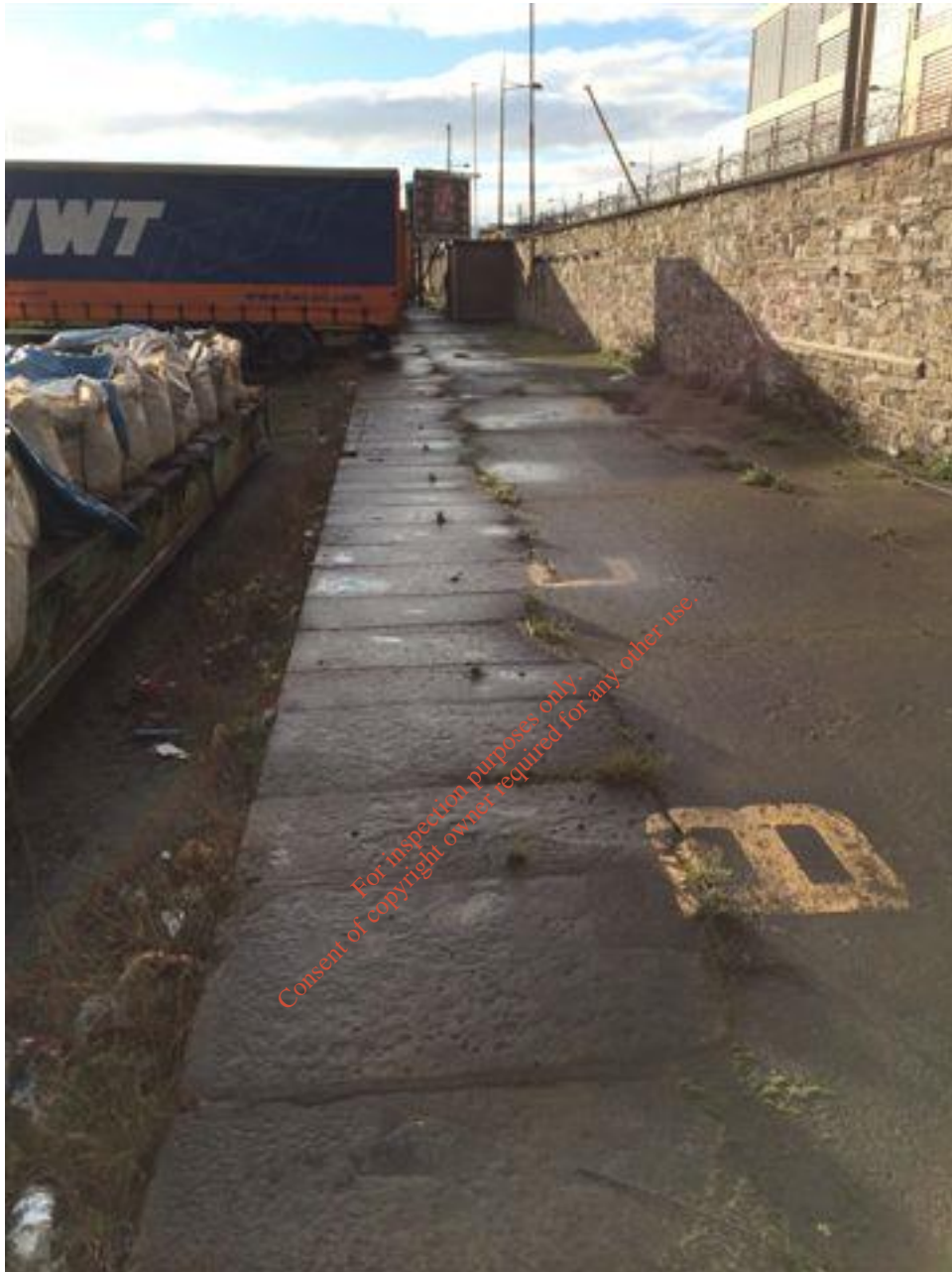
PLATE 10 WESTERN LIMESTONE WALL AND ORIGINAL QUAY WALL ALONG WESTERN BOUNDARY TO BE CONSERVED VEGETATION TREATMENT AND MAINTENANCE POINTING RECOMMENDED
