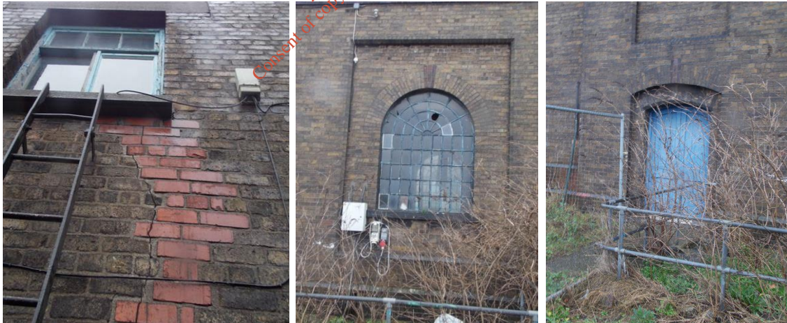
PLATE 17 SHOWING AREAS OF BRICK REPAIR REPAIRS TO IRON WINDOWS AND CONSERVATION AND REDECORATION OF EXTERNAL DOORS
