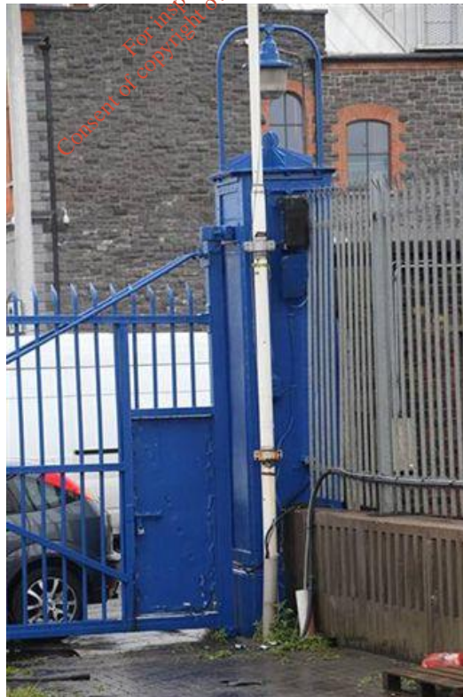
PLATE 9 DETAIL OF RIVETED STEEL GATE POST c 1875
