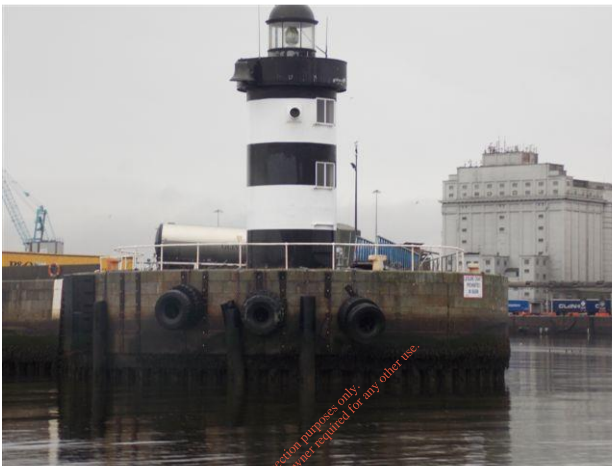
PLATE 6 ORIGINAL 1902 LIGHT HOUSE TO BE RELOCATED ON PIER END WITH 2 COURSES OF CURVED GRANITE BLICKS FORMING A PLINTH THIS WAS MOVED TO THE CURRENT LOCATION IN 1938. THE METHODOLOGY FOR LIFTING IS SHOWN IN APPENDIX 1
