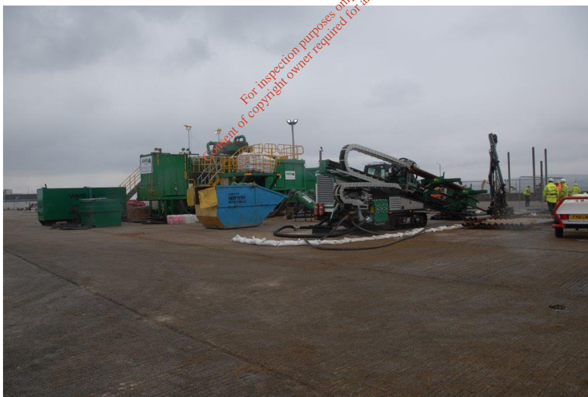
Plate 2: Typical Mud Handling Plant (located to rear of the drilling plant)
