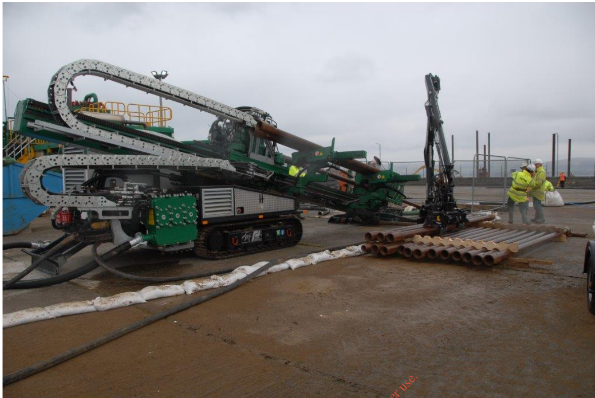
Plate 14.2.1 Typical Horizontal Directional Drilling Rig
