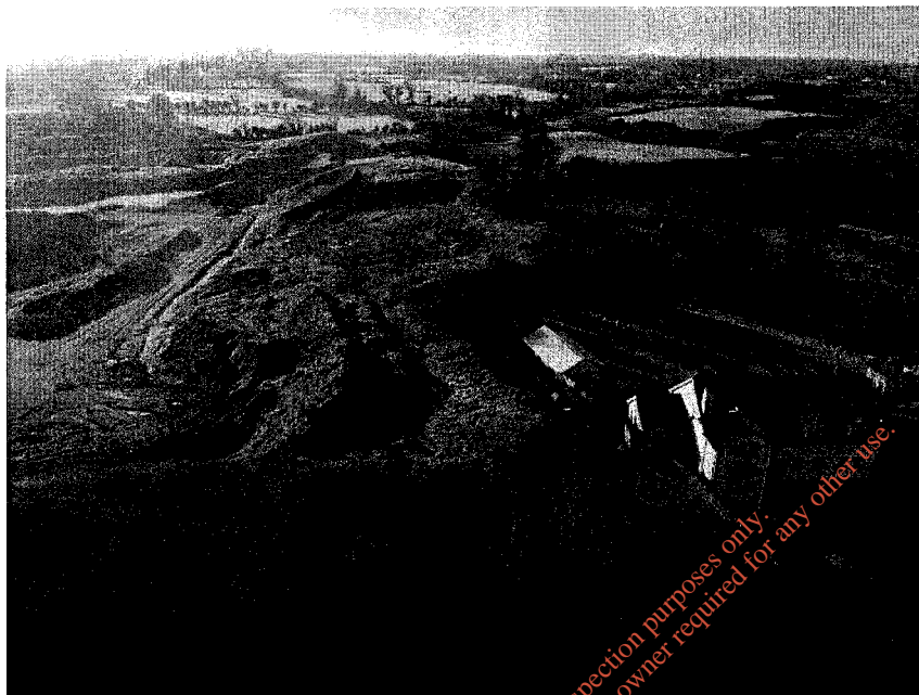
Proximity of Family Home to Ballinderry Pit.
