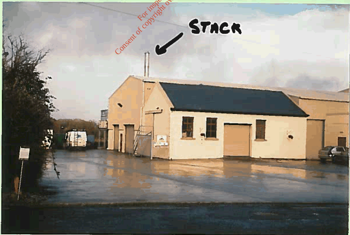
FACORY - OLD CREAMERY BUILDING IN FOREGROUND,
