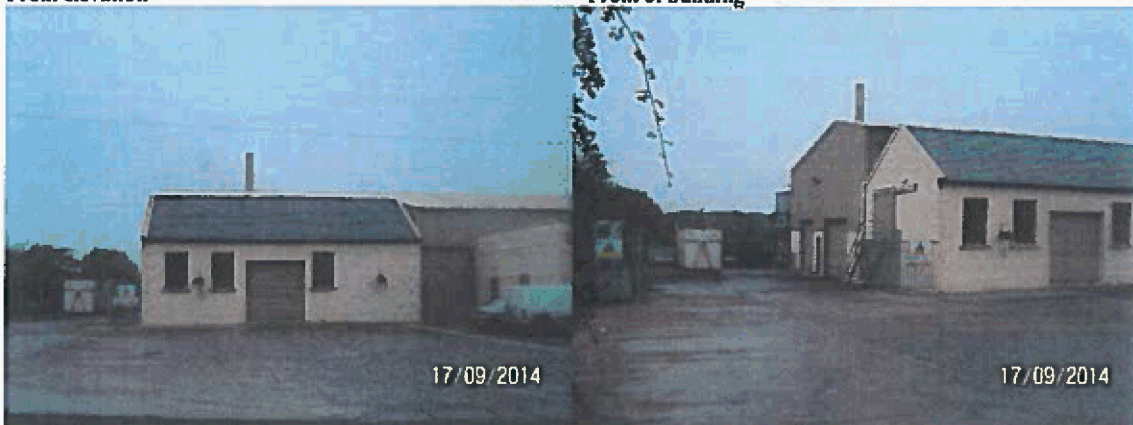
Front of building
