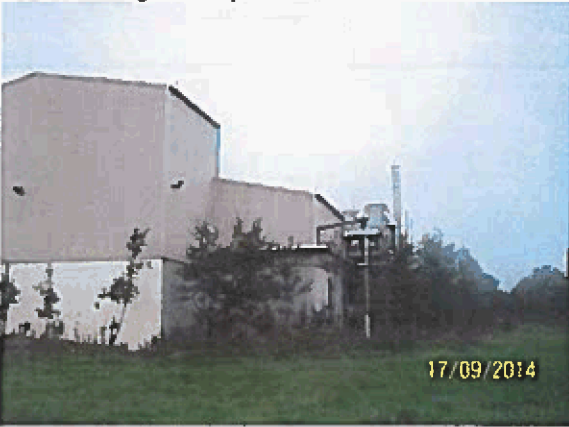
Rear and side of building
