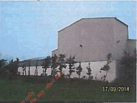
South east side of building
