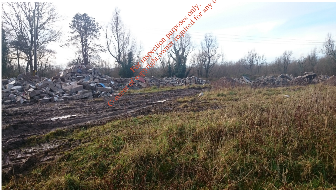
Photo 2 – Concrete Floor from previous slaughtering building (concrete is to be crushed and reused on-site for truck laydown areas).
