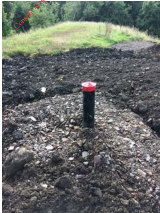
Photograph 2: Groundwater Monitoring Well Installation, The Naul, Clashford, Co. Meath.
