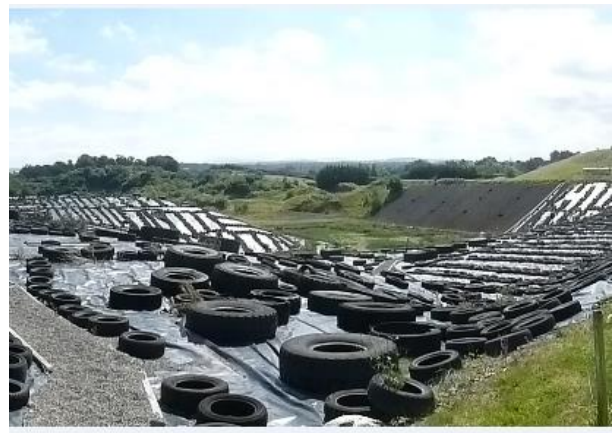
Tyres currently holding down the temporary capping system
