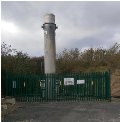
The Existing Landfill Gas Flare
