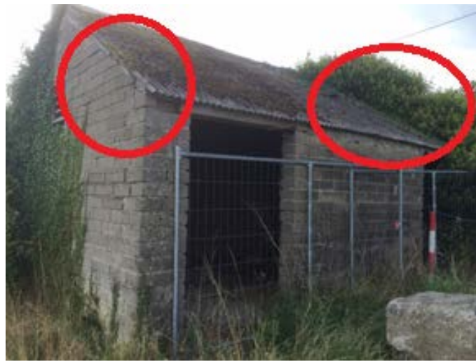
Photo 11.1: Building (shed) with cracks in brick work and dense ivy cover. Point A on Figure 12.2.
