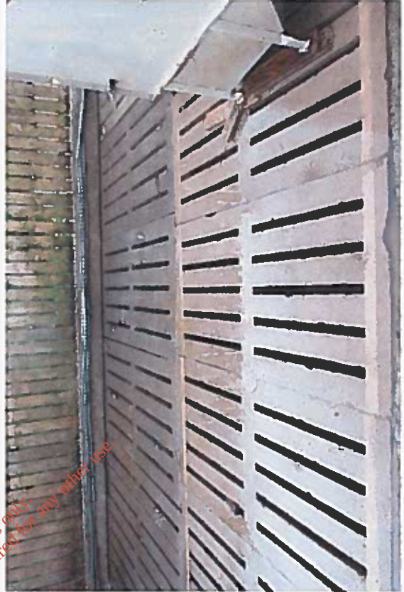
. Attenuation tank for the collection of effluent. Effluent from here is pumped up to the settlement lagoons
