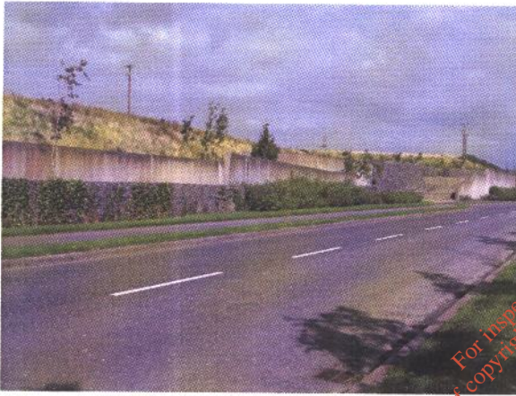
Southern end of site looking east
