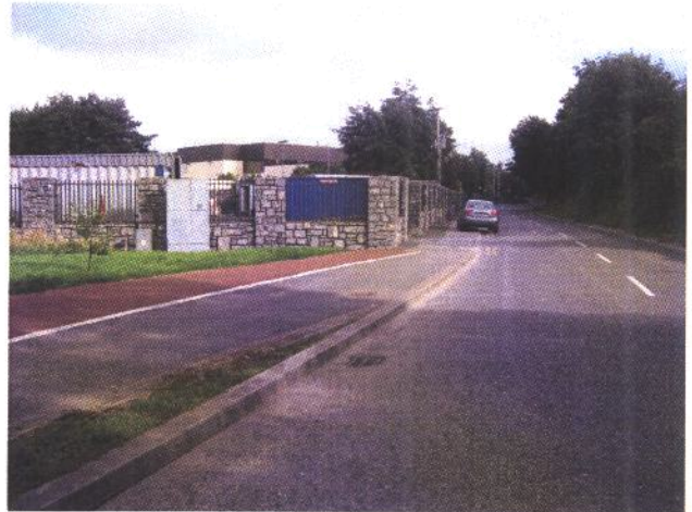
Carrowbeg Road & boundary wall of existing Allergan complex
