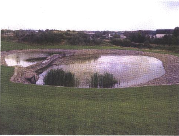
Existing attenuation pond on site
