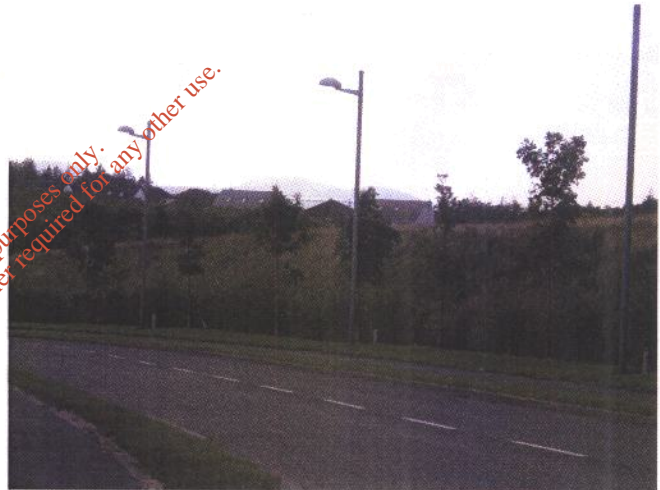
Western site boundary
