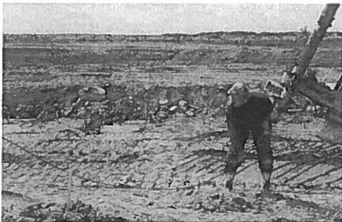
Threading the cable up the drill pipe.
