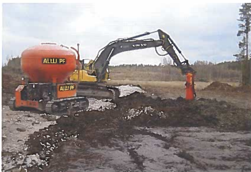
Figure 9 Mass Stabilisation Rig in Operation
