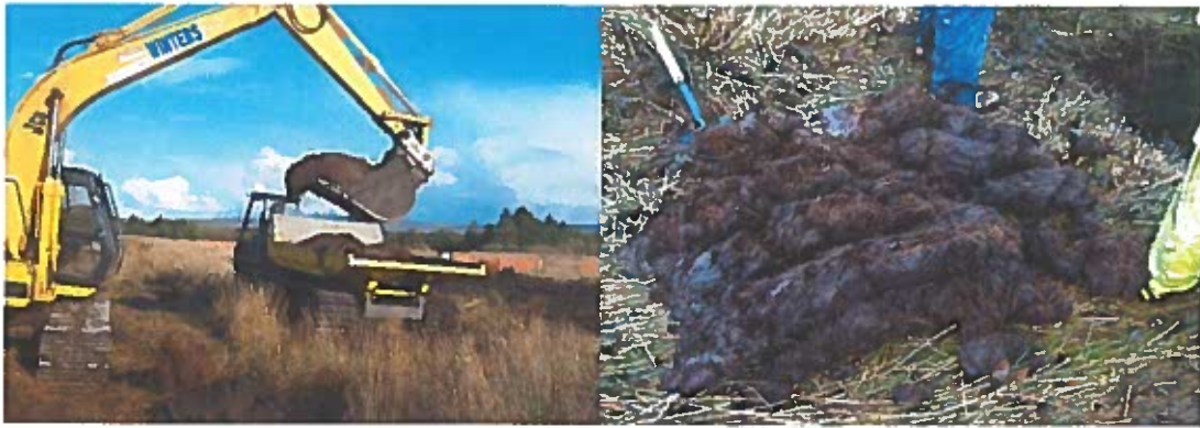
Figure 5 Excavation & Loading of Peat into Tracked Dumper
