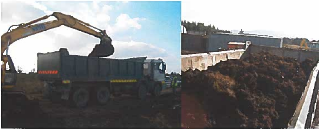
Figure 8 Loading Windrowed Peat into 8 Wheeler Truck & Its Condition after 18km Journey
