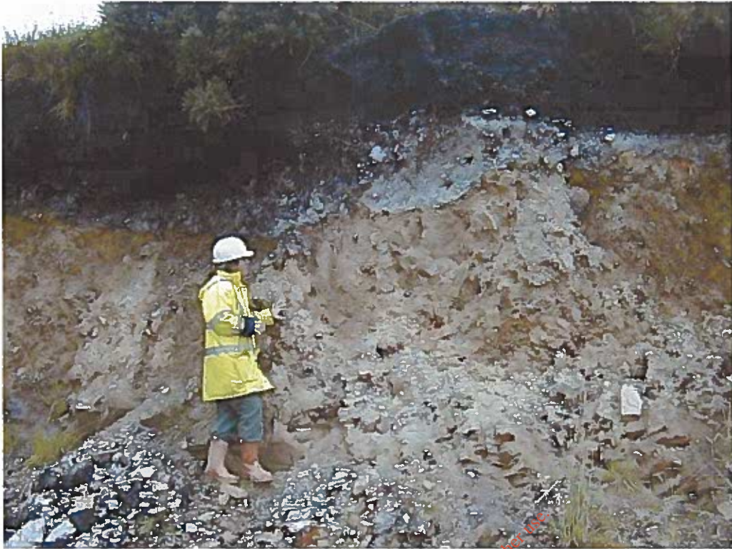
Plate 1. Quarry to east of terminal site, showing peat overlying head. Note light grey leached zone (A horizon) with thin iron pan layer (arrowed) developed at interface with underlying light brown head.
