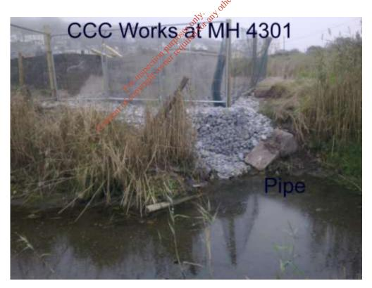
The rocks/rock gabling were placed around the base of the manhole and on top of an open concrete pipe beneath the manhole in the surface water drain beside our property. Cork County Council need to confirm what the function of this pipe is and that there are no connections to the sewer network as the outlet of the pipe is turned and directed toward MH 4301 and the Strand Holding Tank.
