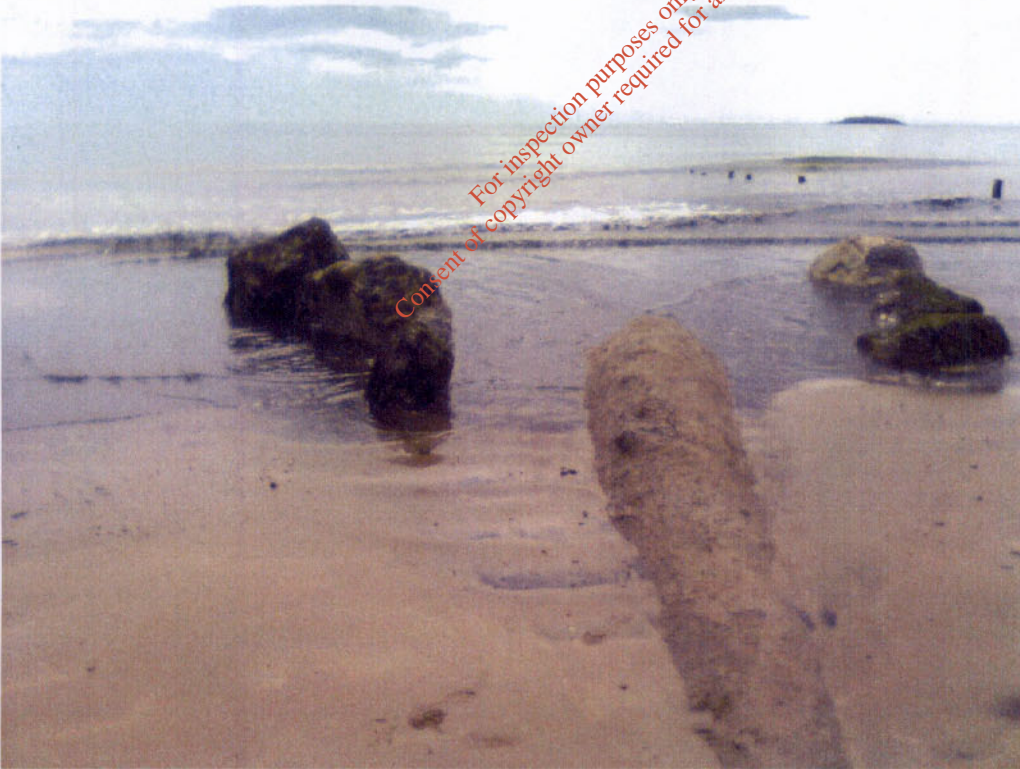
Lower Outfall Extended
