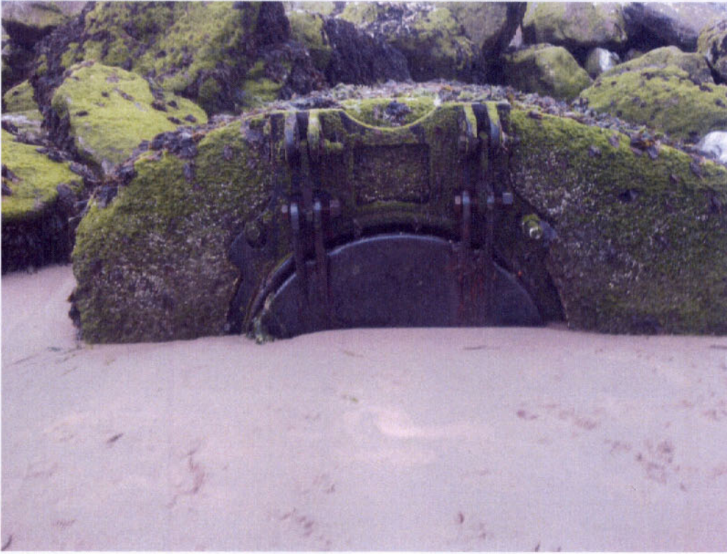
Upper Outfall Buried
