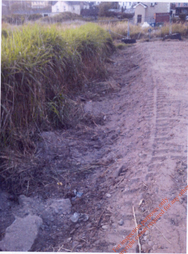
Filling to west of Strand Holding Tank
