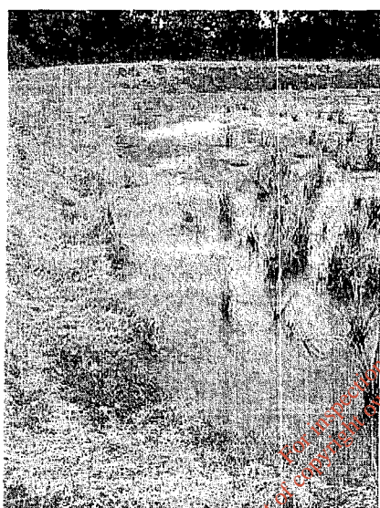
Figure 1. Wetland segment one of constructed wetland system used to treat meat industry wastewaters at Ballon Meats, Co. Carlow.
