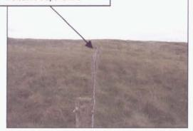
The stock proof fences including timber stakes are inclined in both directions. The sheep wire is extremely taught and deformed to reflect the tension that is imposed on it from the displaced timber stakes. This is evident from a site visit.
