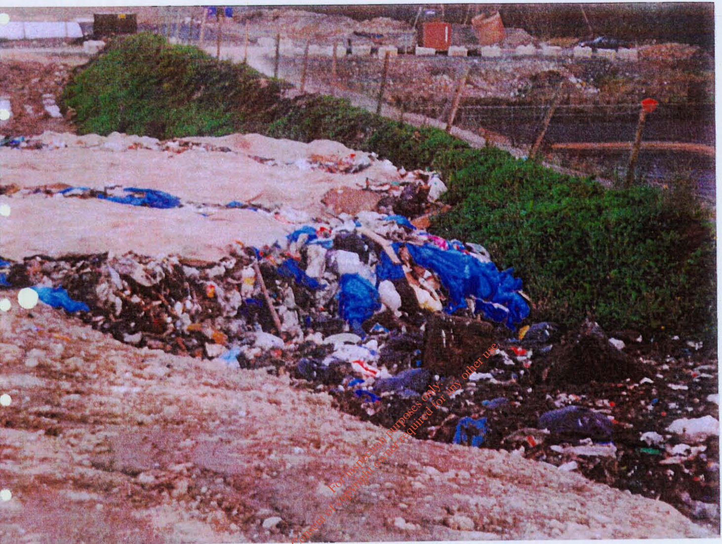
TIP FACE POOR COMPACTION LARGE AREAS UNCOVERED
