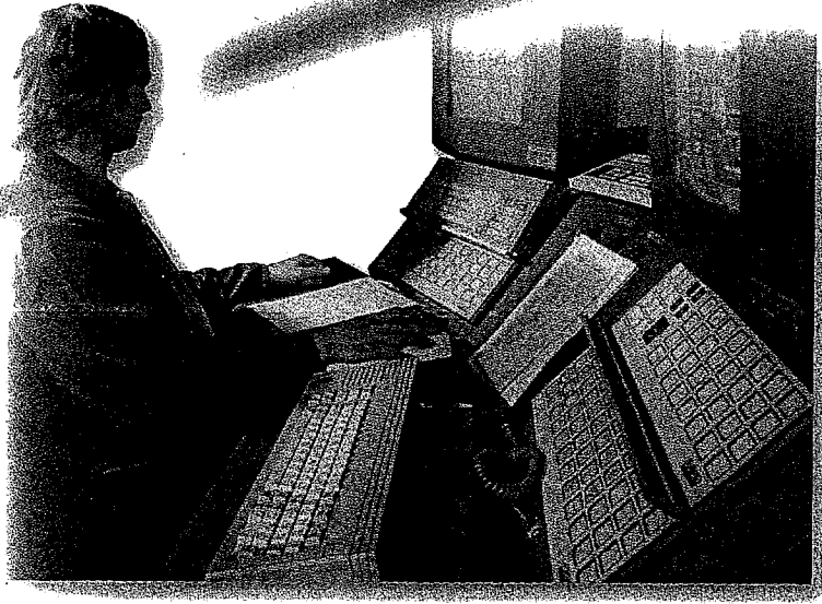
Indaver control room, Waste to Energy plant
